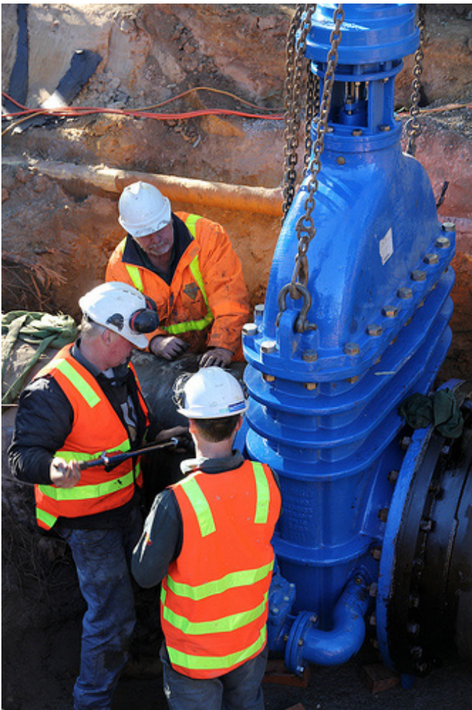
Final installation - AVK Series 54 Gate Valve
