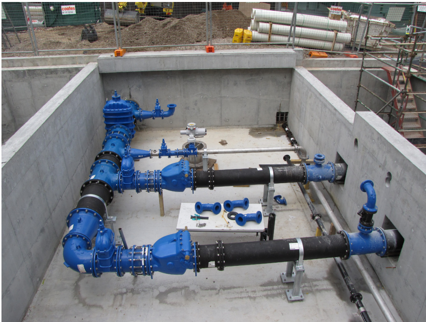
A pit construction at Neutral Bay in the Sydney metropolitan area with the AVK valves being installed
